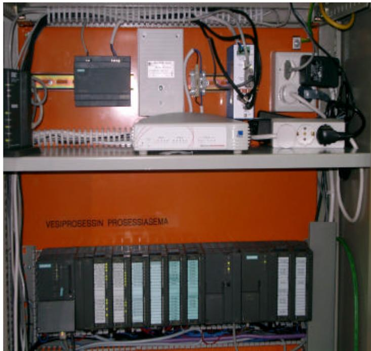
**Figure 3: The main control cabinet of the waterprocess**
